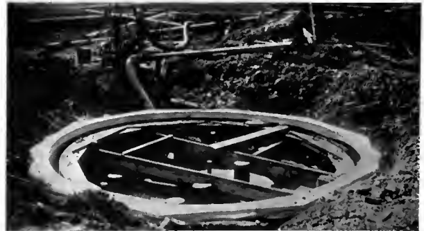
SHOWING TEMPLET AND CENTER STEEL PIN
